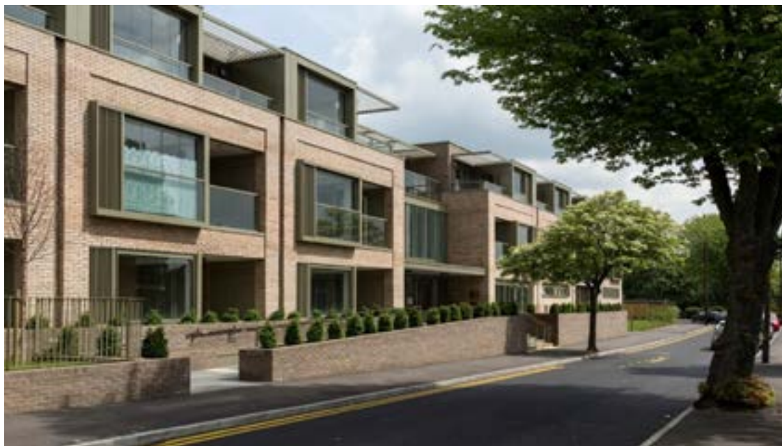
Well-designed and easily identifiable ramped and stepped approach to a communal entrance. (Courtesy of: PRP Architects, Windmill Court, Chingford. - Image © Tim Crocker 2016)
