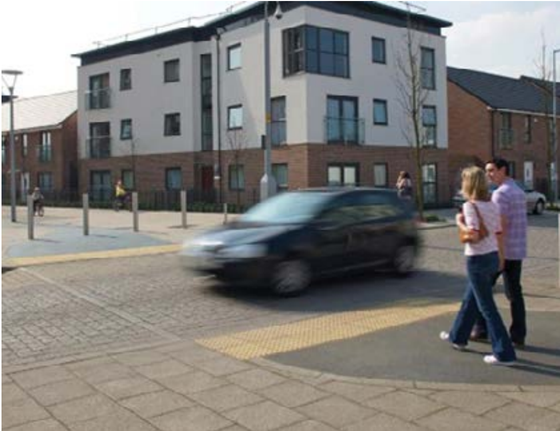
Dropped kerbing and tactile paving helps with safe navigation of outdoor spaces (Courtesy of: Marshalls Landscaping UK)
