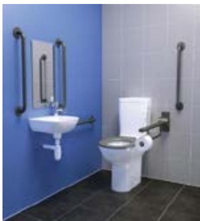
Finished with enhanced contrast between critical elements. (Courtesy of: Armitage Shanks)
