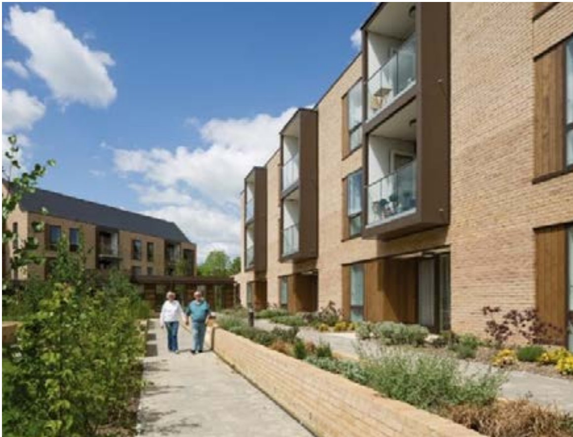
Clear unobstructed footpaths ease navigation Courtesy of: PRP Architects, Farrow Court, Ashford. - Image © Richard Chivers)
