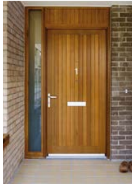
Colour contrasting door ironmongery with clear numbering (Courtesy of: PRP Architects, Windmill Court, Chingford. - Image © Tim Crocker 2016)
