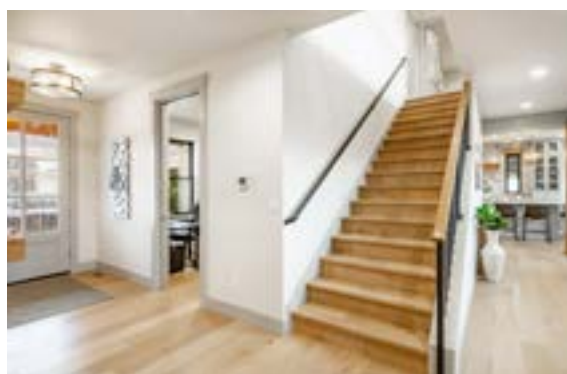
Good width on stairs with contrasting rail. (Courtesy of: Getty Images)
