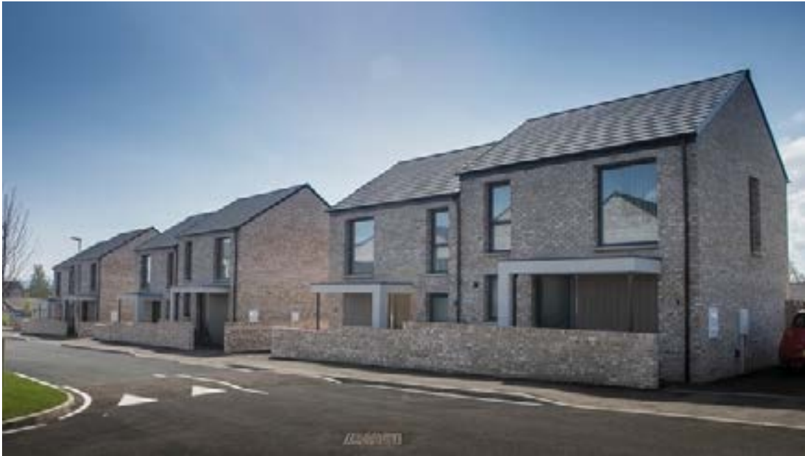
Gardenmore Green Social Housing Scheme. (Courtesy of: Hall Black Douglas Architects)
