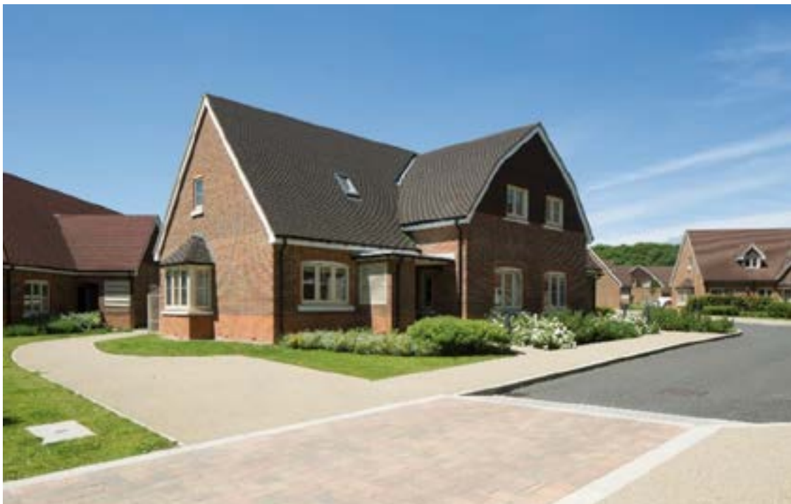
Car parking provides a level approach to the property (Courtesy of: PRP Architects, Durrants Village, Faygate. - Image © Richard Chivers)
