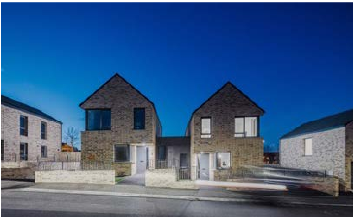
Good external lighting with clearly visible access (Courtesy of: Hall Black Douglas Architects)
